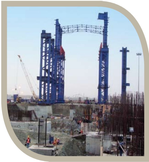
Greenfield expansion at Odisha, India
